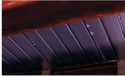
Noggins glued between steelwork flanges.
