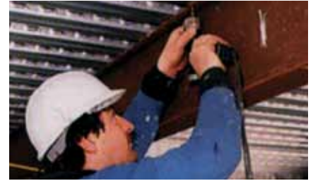
Fixing stud welded pins
